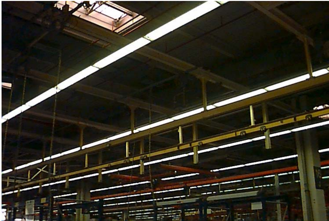
Picture 1: Lighting installation in the assembly hangar
