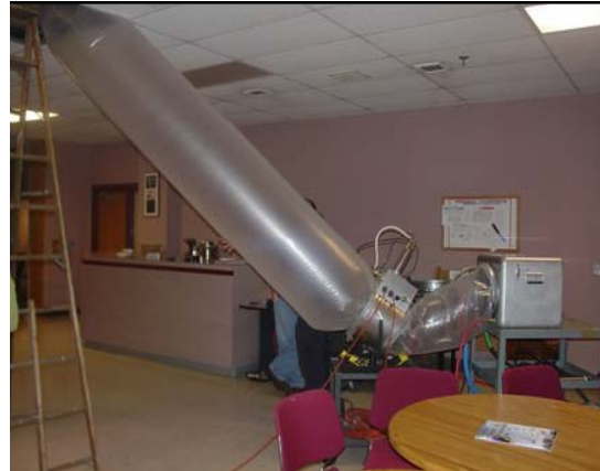
Figure 6 ó DUCT SEALANT SERVICING
